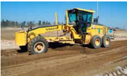
Levelling with a Grader
