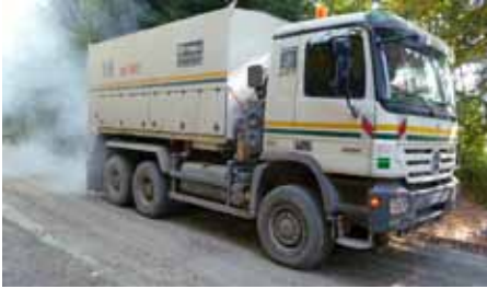
Spreading of cement-NovoCrete®
