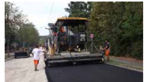
Installation of asphalt after 48h
