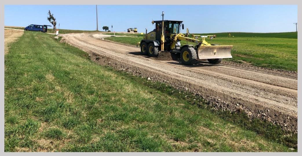
Spreading of the exactly defined amount of cement-NovoCrete® mixture per square meter (m2) and first milling of the mixtrure
