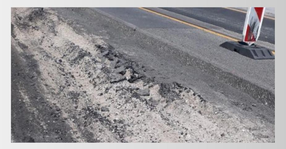
Spreading of the exactly defined amount of cement-NovoCrete® mixture per square meter (m2)
