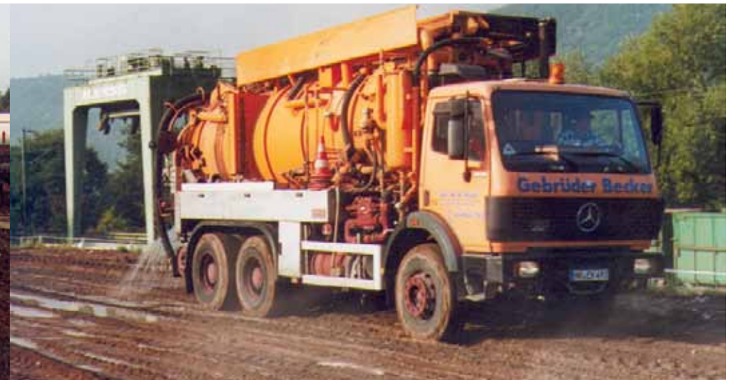
Fig. 3: A pump truck was used to water the base course.
