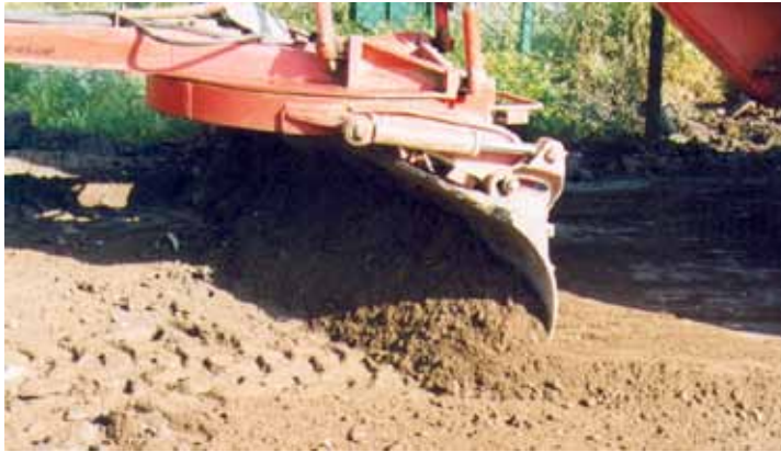
Fig. 5: Immediately after milling in the binder, the base course was dynamically compacted and production of the precise grade layer commenced.
