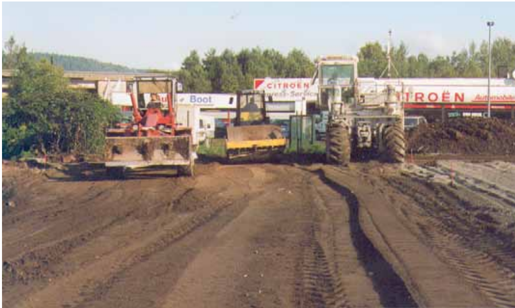
Fig. 5: Immediately after milling in the binder, the base course was dynamically compacted and production of the precise grade layer commenced.
